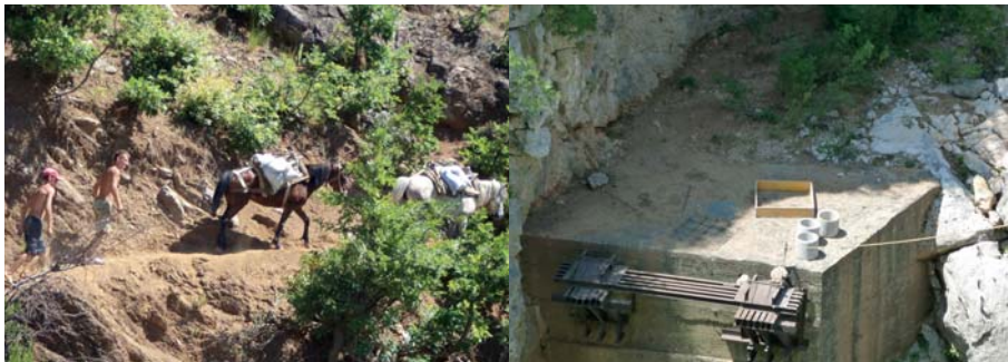
Figure 6. Transport of construction material, Mules, improvised cable cars.
