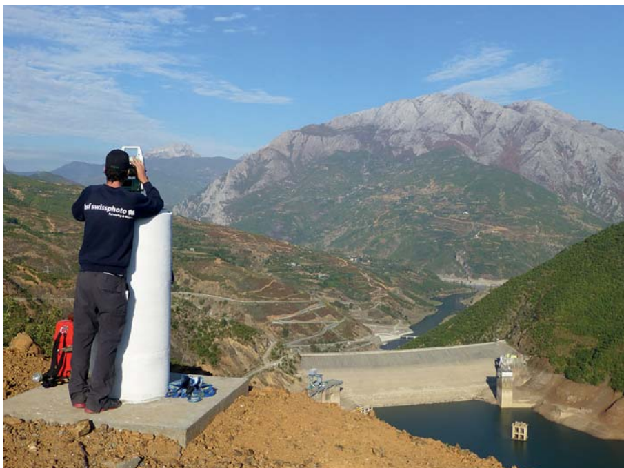
Figure 1. Geodetic Monitoring at Fierza HPP.
