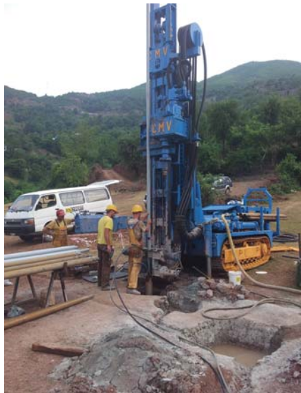
Figure 3. Drilling works for inclinometers with sub-contractors Altea Geostudio2000 at Porava.
