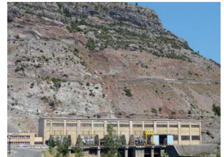
Figure 7. Powerhouse in Koman with land slide area in the background.
